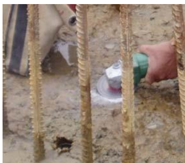
Figure 3.26 Clean the Pile Head
